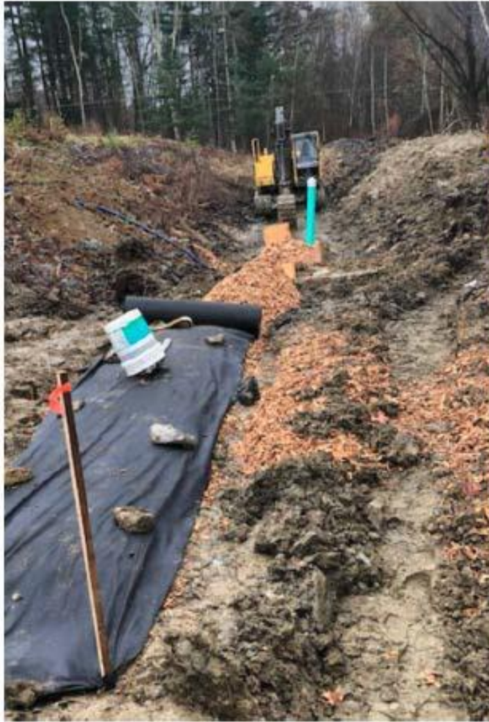
During PRB Installation
