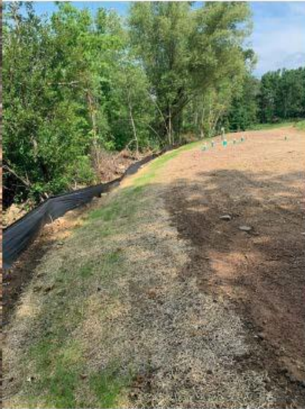
PRB after construction completion
